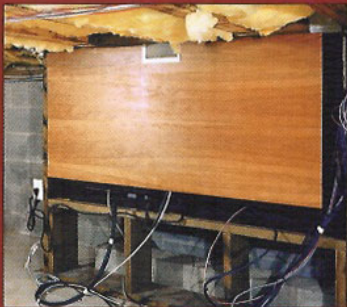
To mobilize the plasma, EDG called on Electrokinetics to build a double rack-and-pinion lift to support the display and center-channel speaker
